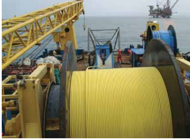
► Coiled line pipe S-Laid from a DP vessel (left), and Coiled Line Pipe laid as piggy back from a DL barge. (right)
